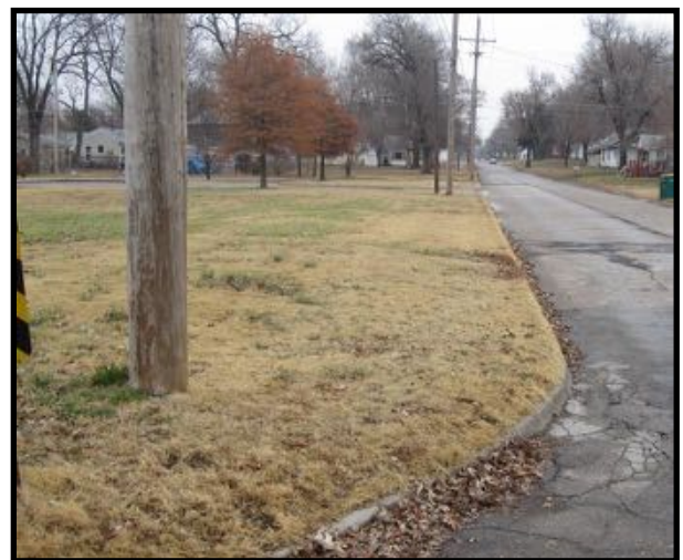
Stretch of NW Paramore St. from NW Central St. to N Kansas Ave. with no sidewalks, one of the main walking routes to and from school
