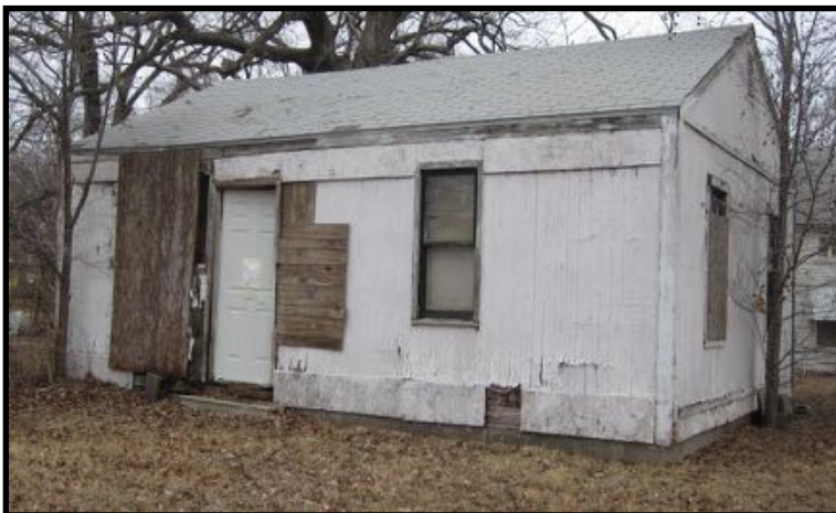
An abandoned house (807 NW Gordon St.) where stray dogs were coming in and out of the structure
