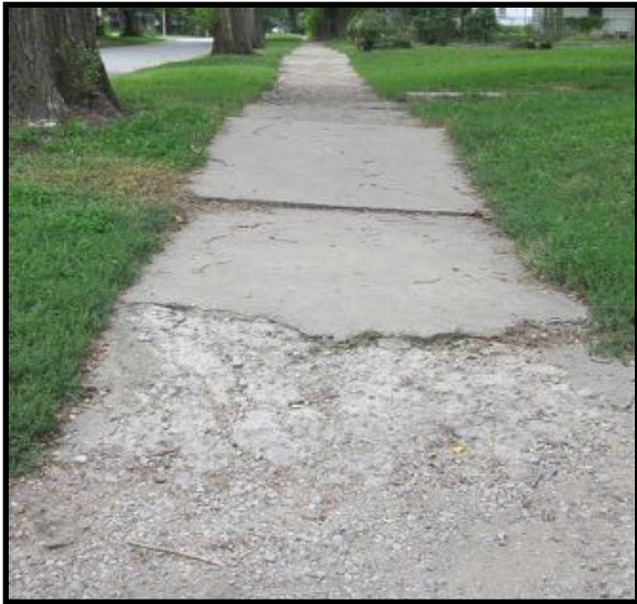
Crumbling and raised sidewalk along NE Monroe St., less than a block away from Quincy Elementary
