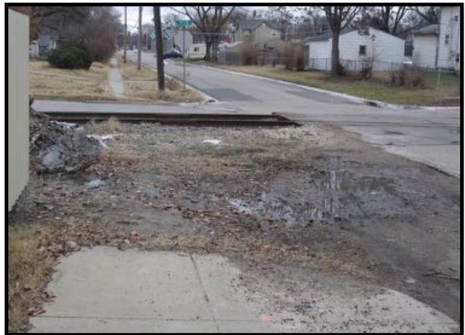
End of sidewalk before railroad crossing at NW Tyler St. and NW Morse St. forcing pedestrians to cross in the street
