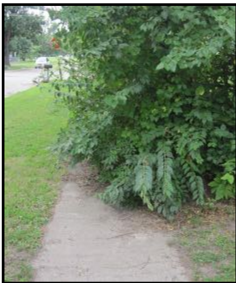
Overgrown weeds covering sidewalk on NW Harrison St., N of Paramore St.
