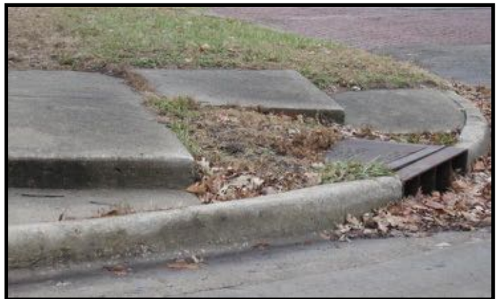
Lack of access ramps at SE corner of NW Jackson St. and NW Grant St. with overgrown sidewalks
